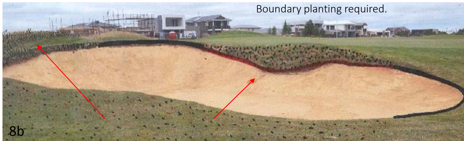
8b; Greenside Bunker, The tongue of the bunker needs to be trimmed slightly. Slight rough should be left on the tongue and also to be top dressed. The walk in and playing area will have a clean edge. The back left shoulder of the bunker to transition into rough grasses .
